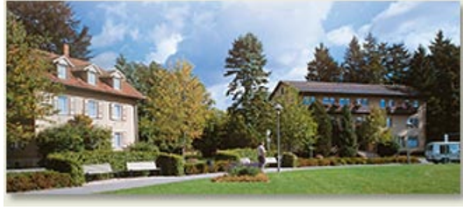
Figure 7. Kursanatorium Karolushaus, Bad Dürrhein. The two buildings above became the clinic known as Karolushaus. Pension Rheiner is at left; Villa Homestead is at right (Undated photograph from Bad Duerrheim website).
