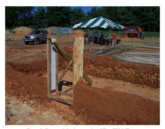
Figure 8. Formwork for door opening of First Wife's House.
