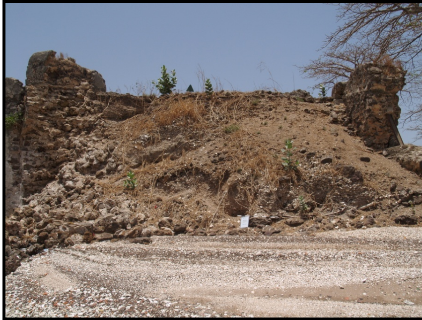
Figure 10. Collapsed north wall of the northwest bastion (photograph by author).
