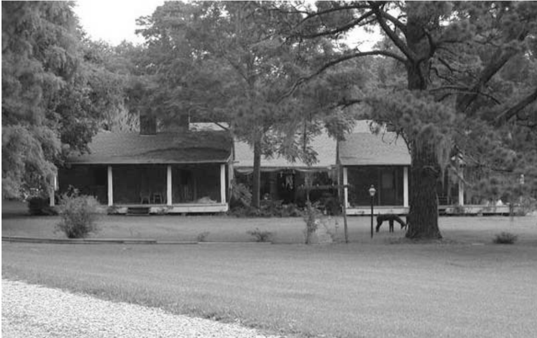
Figure 2. Standing brick structures on Marsh House Slave Quarters site (Image by Jim Delahoussaye).
